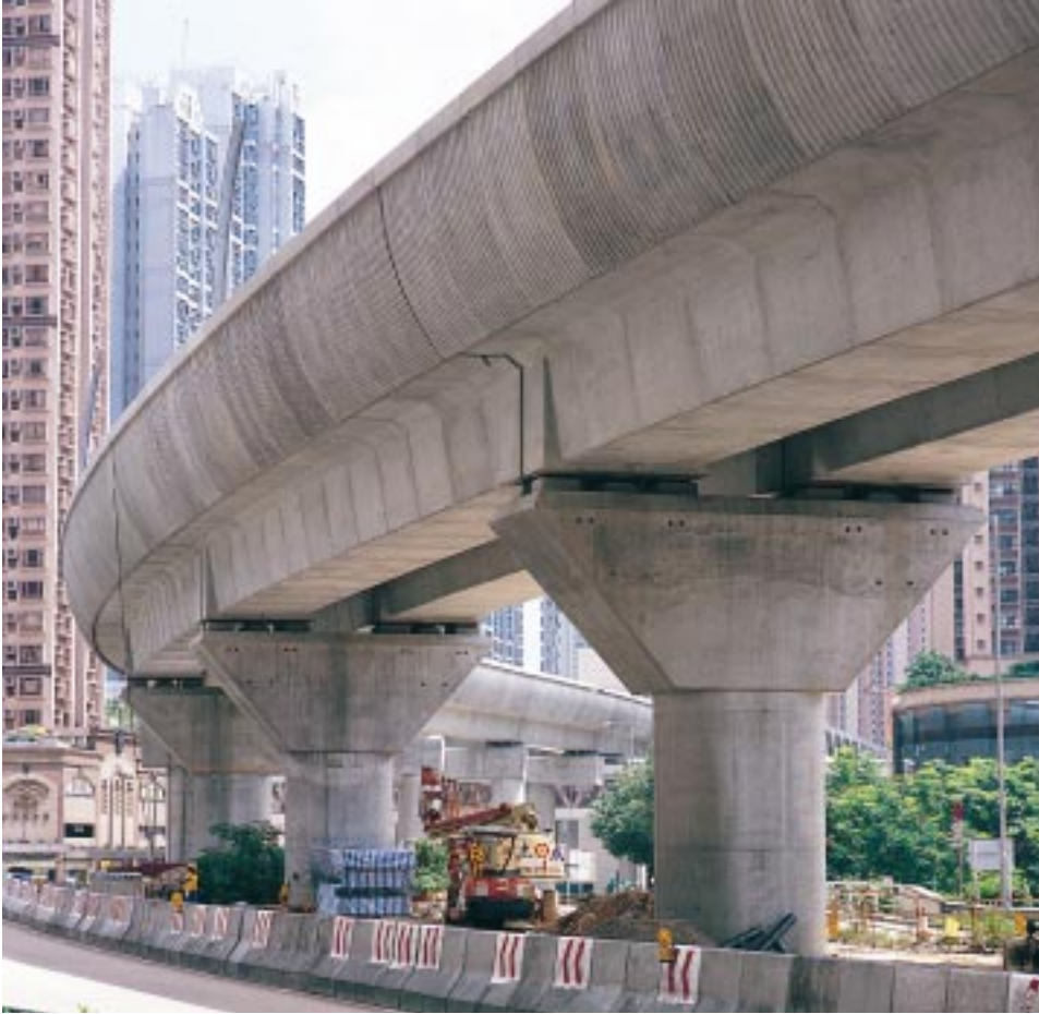
KCRC East Rail Matchcast viaduct segments for this railway project.
