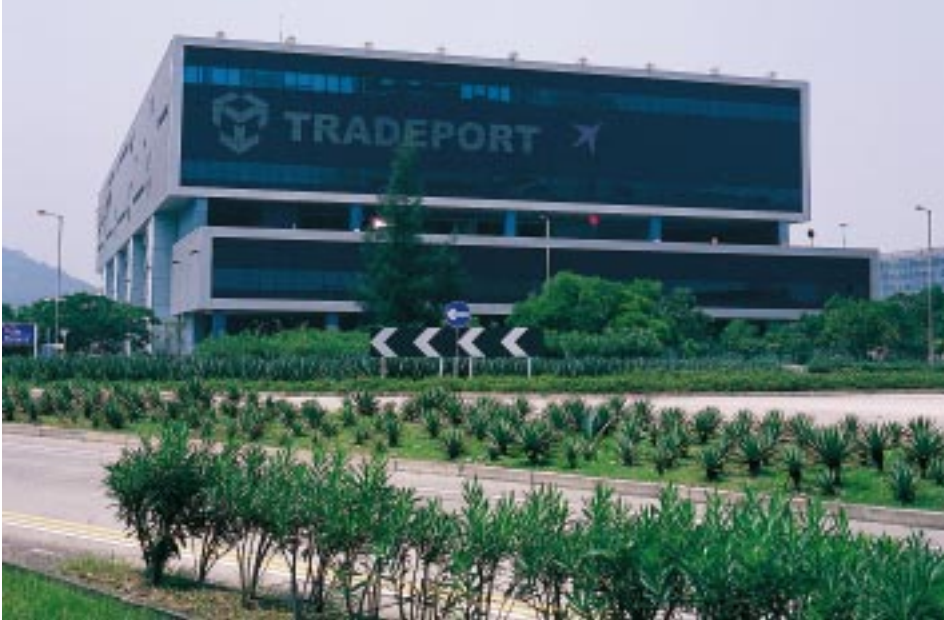
Tradeport Logistic Centre, Hong Kong International Airport Logistics facility at Chek lap Kok airport, Hong Kong, featuring architectural precast concrete used as permanent formwork.
