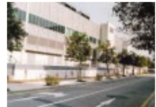
Tradeport Logistic Centre, Hong Kong International Airport Logistics facility at Chek lap Kok airport, Hong Kong, featuring architectural precast concrete used as permanent formwork.
